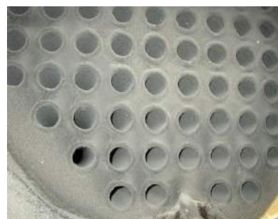
Figure 4-19: Fire-tube boiler (opened) [87]
